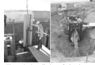
Figure 1. Installation of e-barrier through a plume containing RDX, 2,4,6-TNT, 2,4-DNT and 1,3,5-TNB
